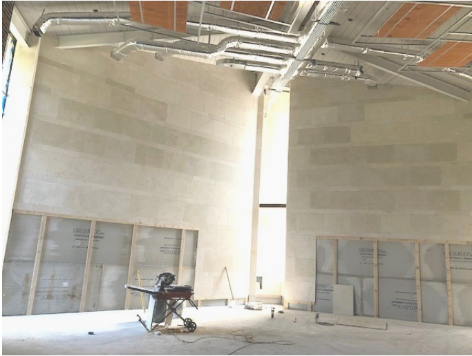
Sanctuary wall with Jerusalem stone installed.
