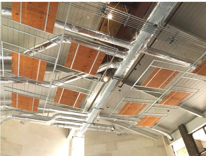
Sanctuary ceiling in progress
